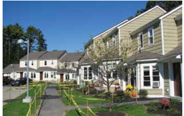
Affordable housing for elders, Boothbay Harbor, 2012
