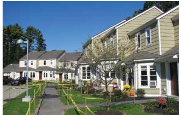
Affordable housing for elders, Boothbay Harbor, 2012
