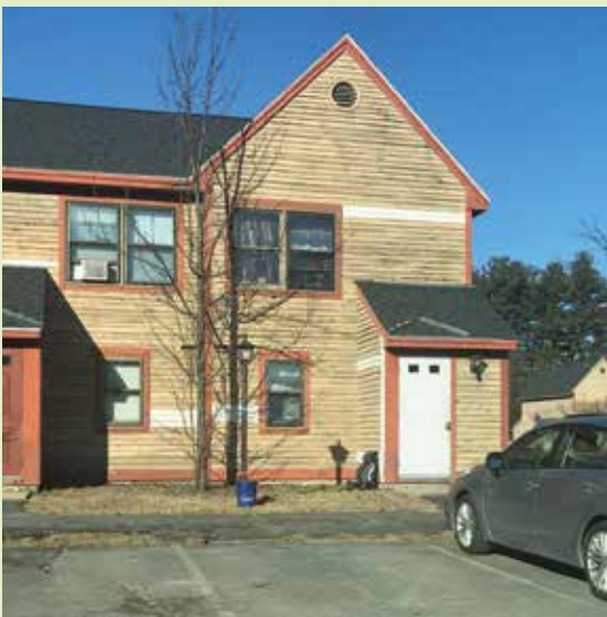
Prior to renovation, Breary Farms, above, was showing its 30 years of age, and was clearly in need of major repairs and upgrades.
