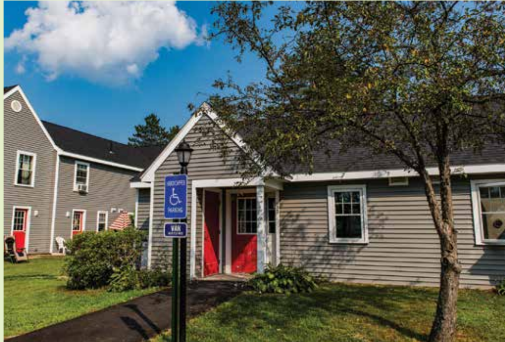
Upgrades at Sanford's Breary Farms included designated units tailored to the needs of people with disabilities.
